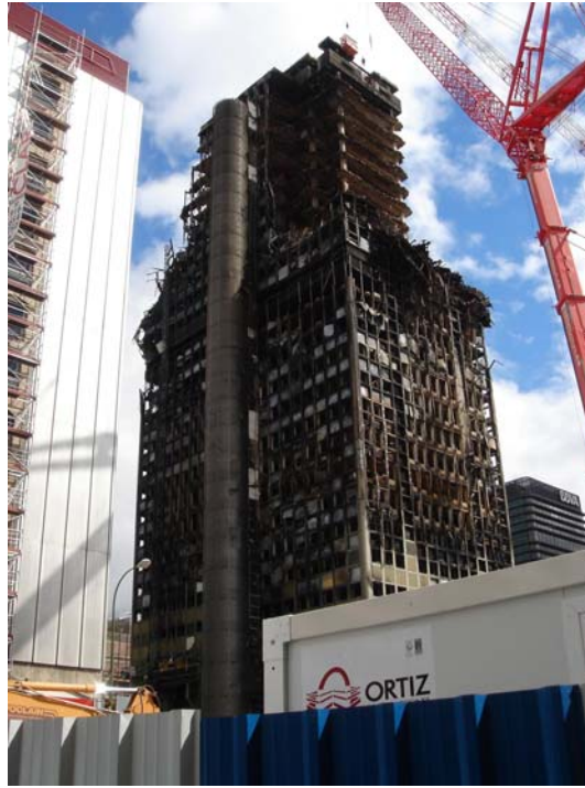
Figure 1. Collapse in the Windsor Building fire
