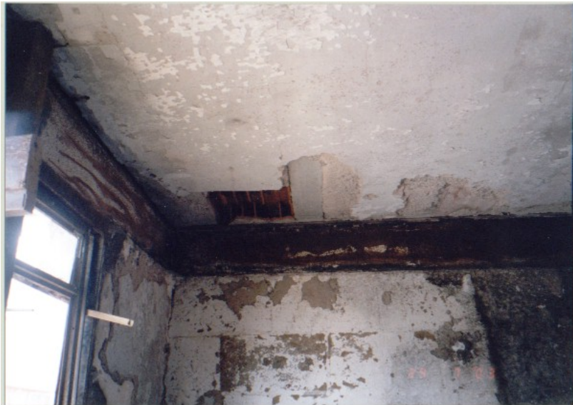
The composite slab started to degrade just close were the fire initiated
