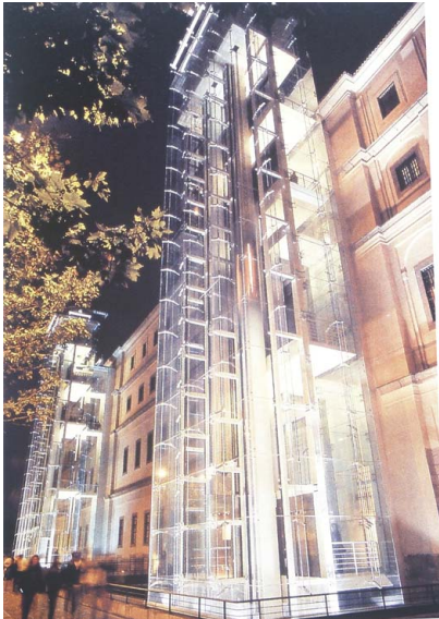
Fig.10 Glass service Tower / Madrid
