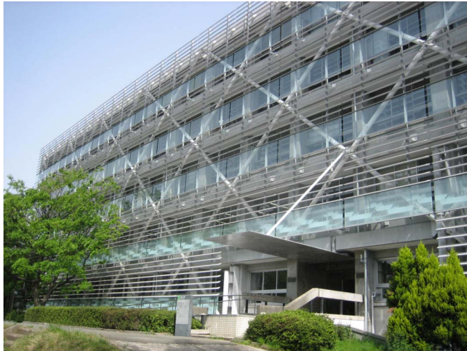
Fig.17 Building Façade after the Retrofit
