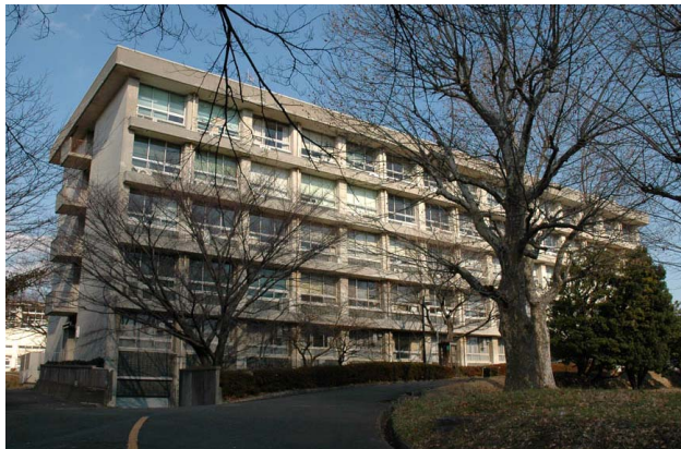
Fig.15 Aged Building before Seismic Retrofit
