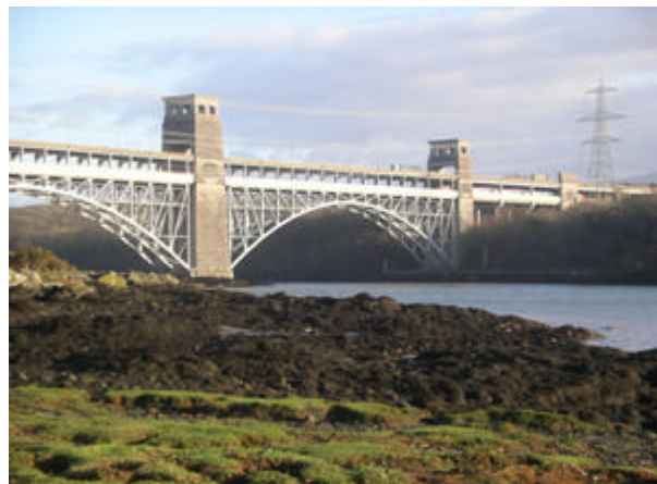
(b). The post 1970 Bridge retains Stephenson's Original Piers [6].
