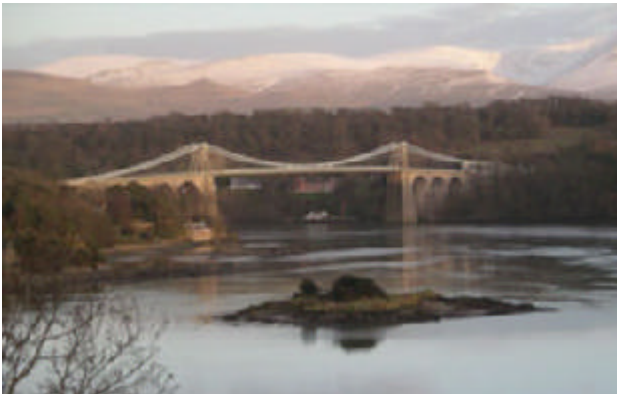
Figure 2. The Menai Suspension Bridge [5].
