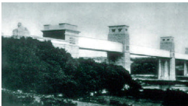
(a). Original box section, in a circa 1852 illustration [2]. Courtesy of Kozai Club.
