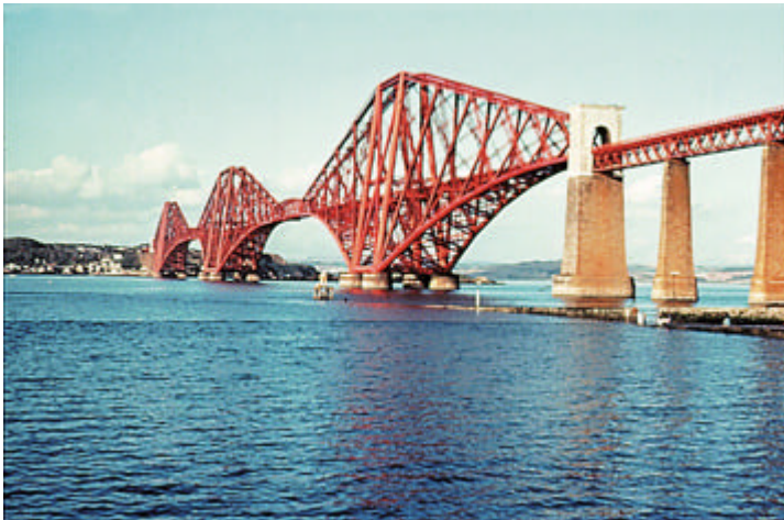
Figure 7. Firth of Forth Bridge [2]. Courtesy of Kozai Club.
