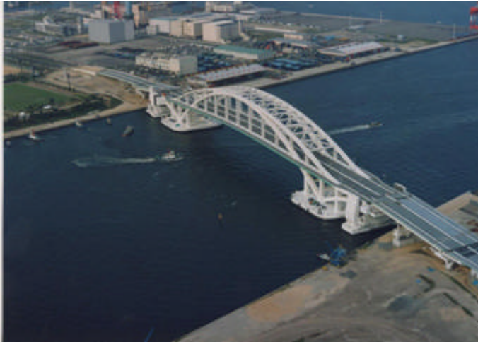
Figure 12. Yumemai Floating Bridge after the on-site installation. Courtesy of Osaka Construction Industry Times.
