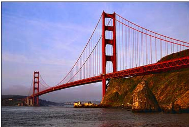
Figure 9. Golden Gate Bridge, San Francisco and Sausalito, California [11]
